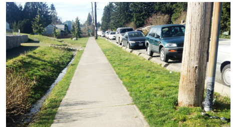
At-grade concrete walkway with wheel stop delineators
