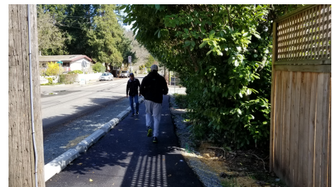
At-grade asphalt walkway
